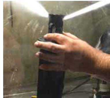
Sprinklers are Tested
